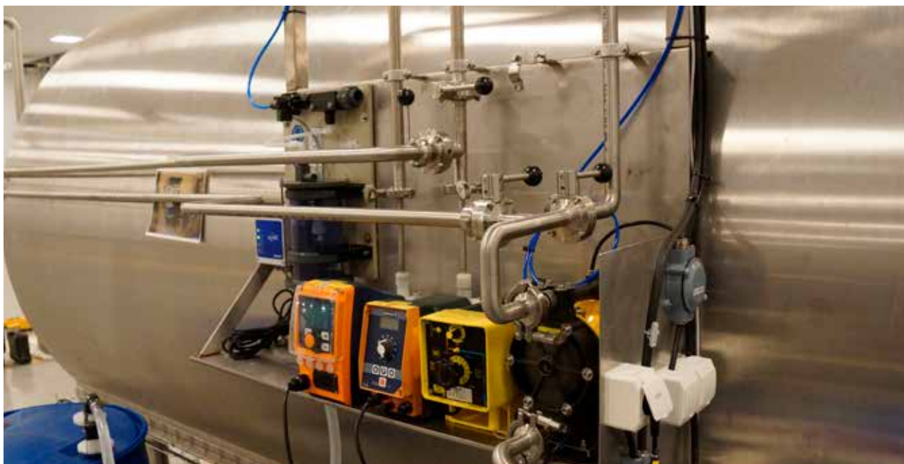
Dosing pumps CIP Wellnox
